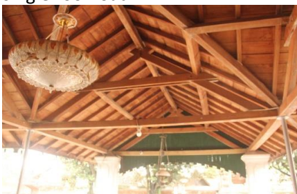
Picture 6 Sawbuck of limasan roof
