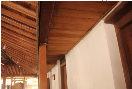
Picture 5 Connection of Tajug and Limasan roof
