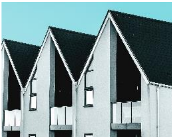
Picture 7. The roof of the house
