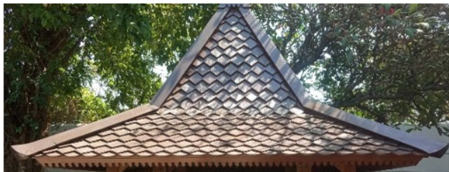
Figure 6. The shape of the Pendopo Rante Sirap is a combination of rectangular pyramids and truncated rectangular pyramids
